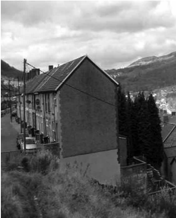
Figure 14 Low carbon retrofit project in Penrhwi-ceiber, Wales
